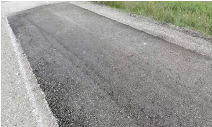
Final result after compaction
