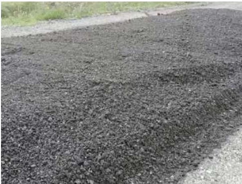
The cold mix after milling and mixing with rejuvenator
